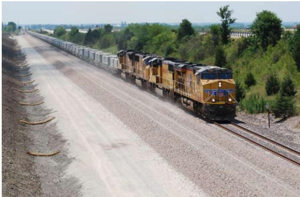
A freight train carrying concrete rail ties travels north on Union Pacific's Chicago–St. Louis line near Odell, Illinois, on a section of track between Dwight and Pontiac where Amtrak trains now travel 110 mph. It features an entirely new railbed, track, and concrete ties. This photo also shows a new siding, which is in the process of being reconstructed to 110-mph standards, 20 feet on center from the mainline.
