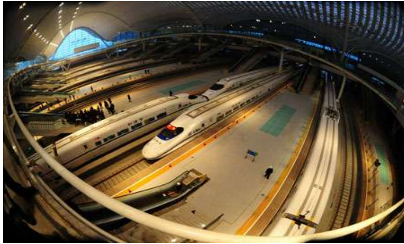
Figure 4. The new Wuhan CRH Station, China.
